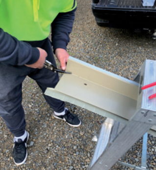
Get work up of the ground
