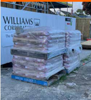
Keep material off the ground
