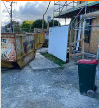
Placing of waste bins
